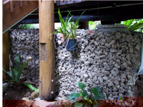
Dry-rock wall to avoid erosion under the walk-way
